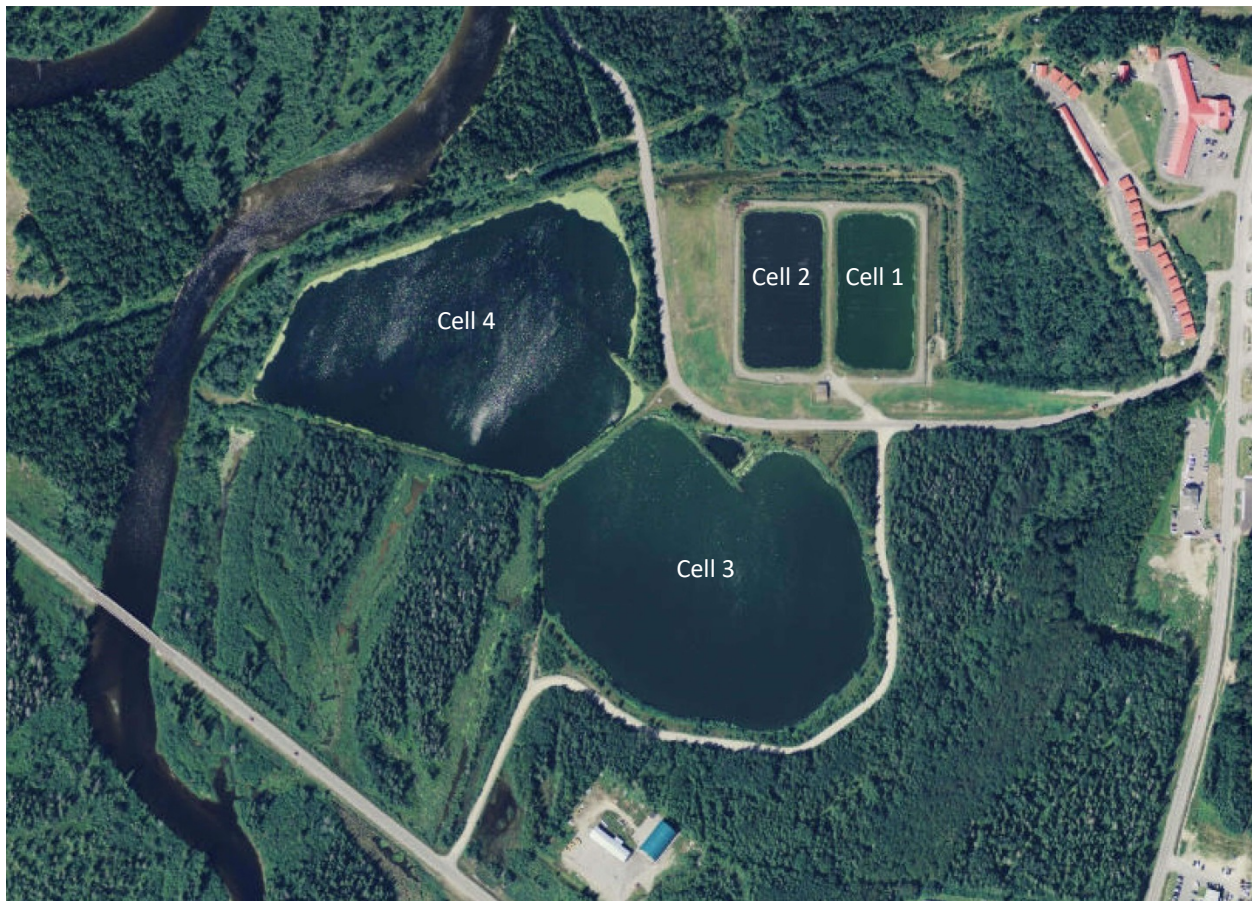
Figure 1: Wawa Sewage Treatment Facility Aerial Photo
