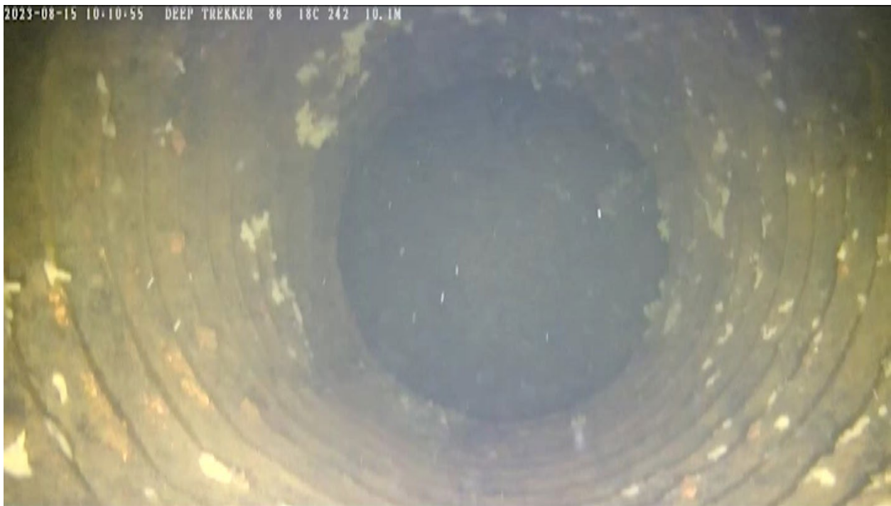
Photograph 5: 90° Section at Duty Intake Structure
