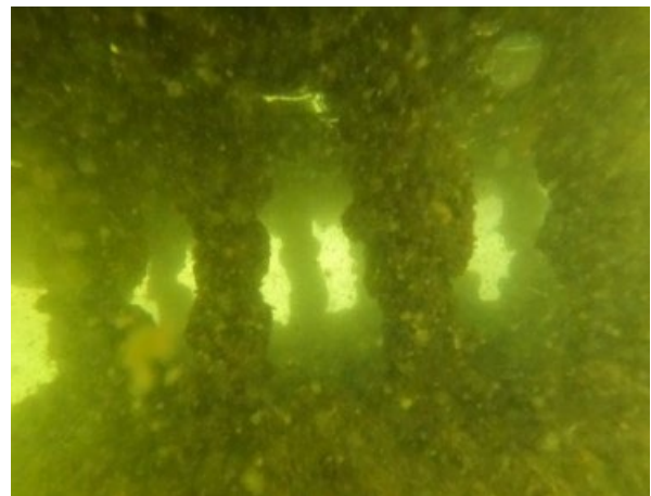
Photograph 2: Marine and Zebra Mussel Growth on Emergency Intake Bar Screen
